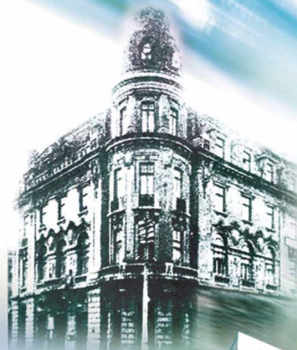
The building of Sofia Commercial and Industrial Chamber 2 Slavianska Str., Sofia built in 1914
