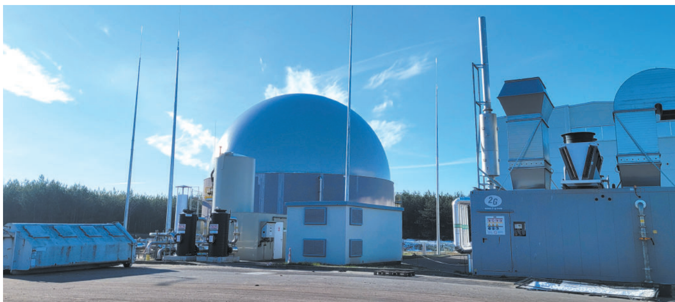
ZUOK "Orli Staw" – digestate and biogas tank, cogeneration unit
